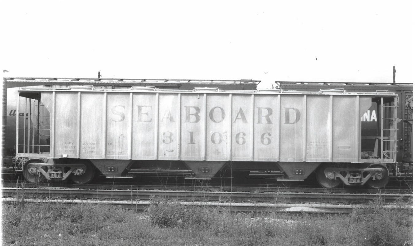
SAL 31066, is seen Atlanta, Georgia on April 30, 1966. The lettering is partially obscured by the spilled lading, which is likely the result of cement or dry rock phosphate. The car was painted a medium gray color and lettered with black stenciling. (C.L. Goolsby photograph, Author's collection)
