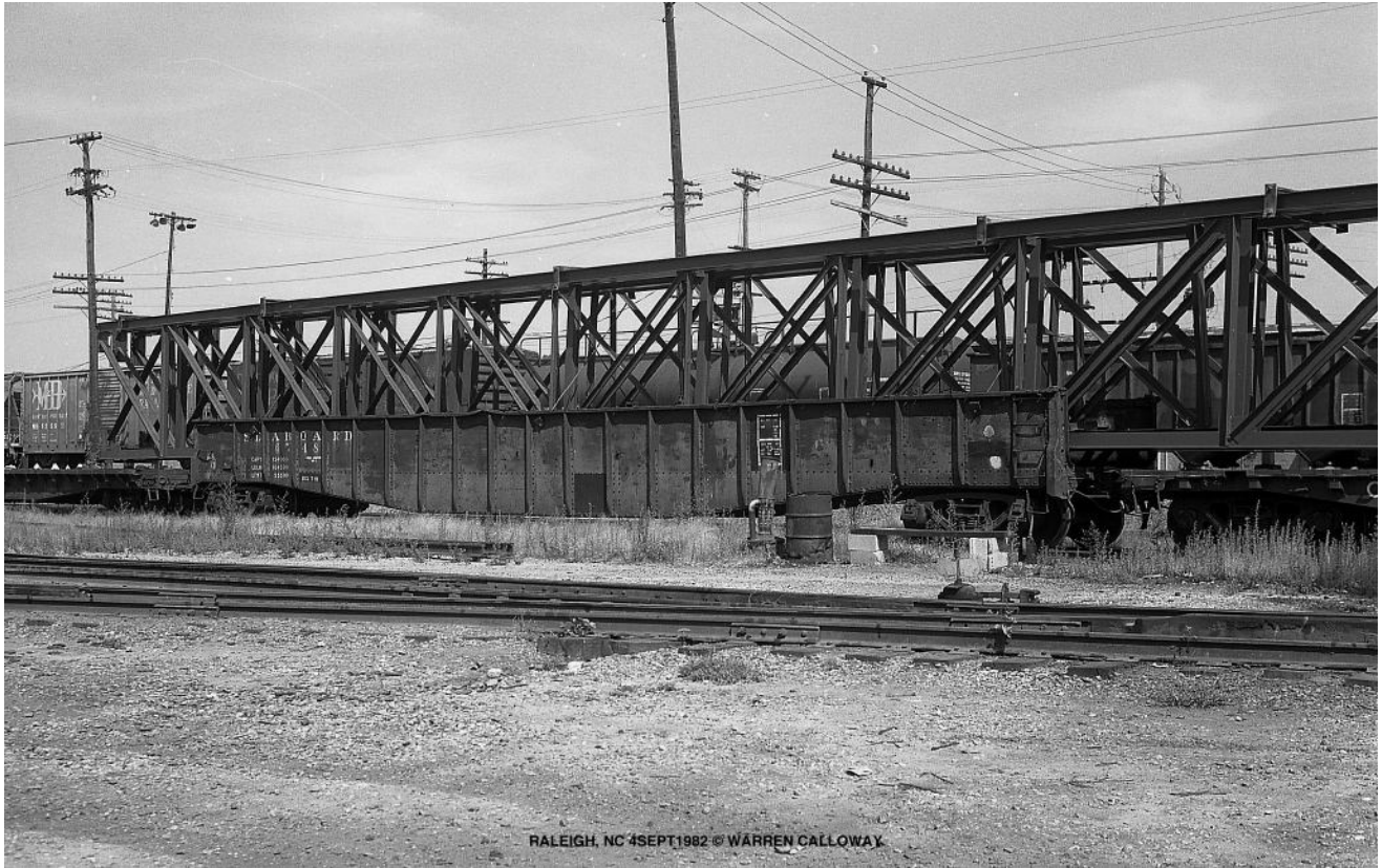
SAL 6548 is loaded with a high and wide load these gondolas were specially designed to handle. The use of idler flats on either side was typical when making special movements of freight. The car was photographed in Raleigh, NC on 09/04/1982. (Warren Calloway photograph)
