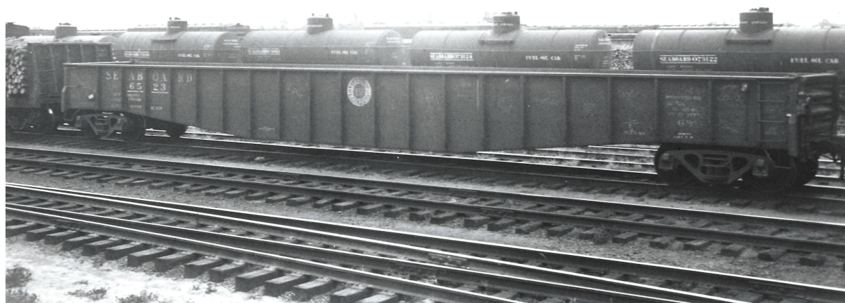
SAL 6523, the most photographed example of all Seaboard GB class gondolas is seen passing through Hamlet, NC. The repack data denotes it was last serviced in 1952. (Col Chet McCoid photograph, Bob's Photo)
